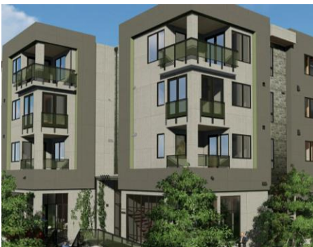
Under Construction: 10300 San Pablo Ave.
