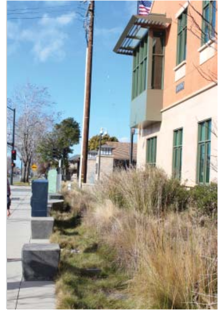
Figure 11. Rain gardens at City Hall
